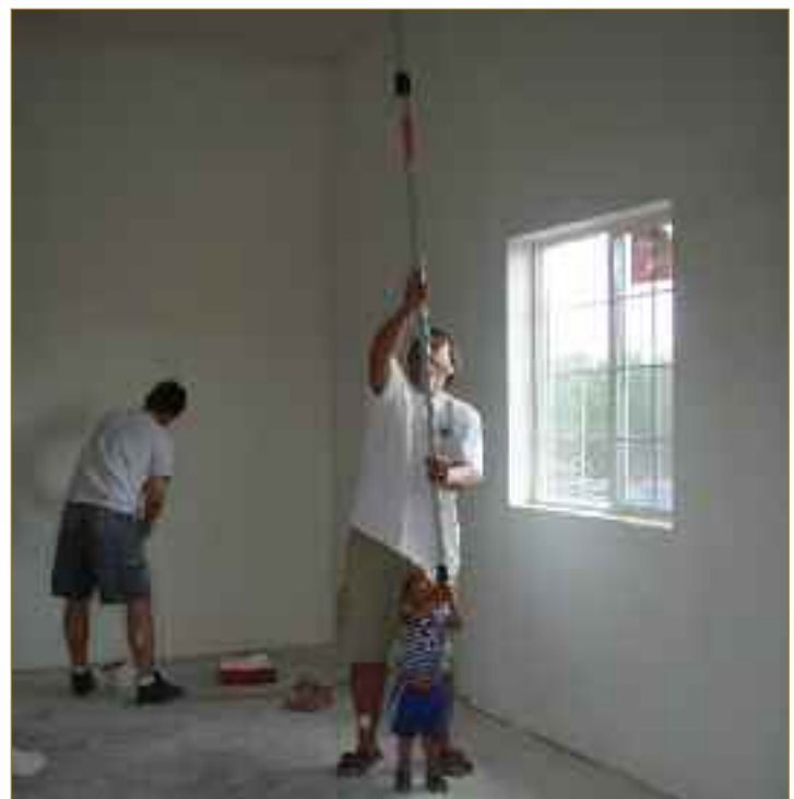
Dameon teaches Greg the proper way to paint ceiling.
